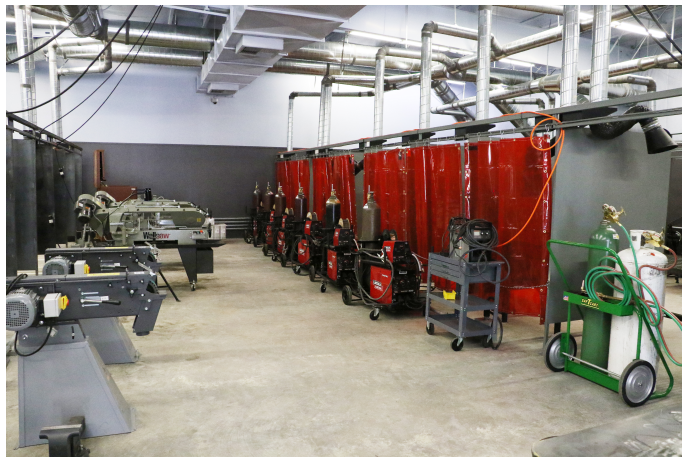
New state-of-the-art welding equipment and specialized welding booths have been installed with a custom ventilation system.
